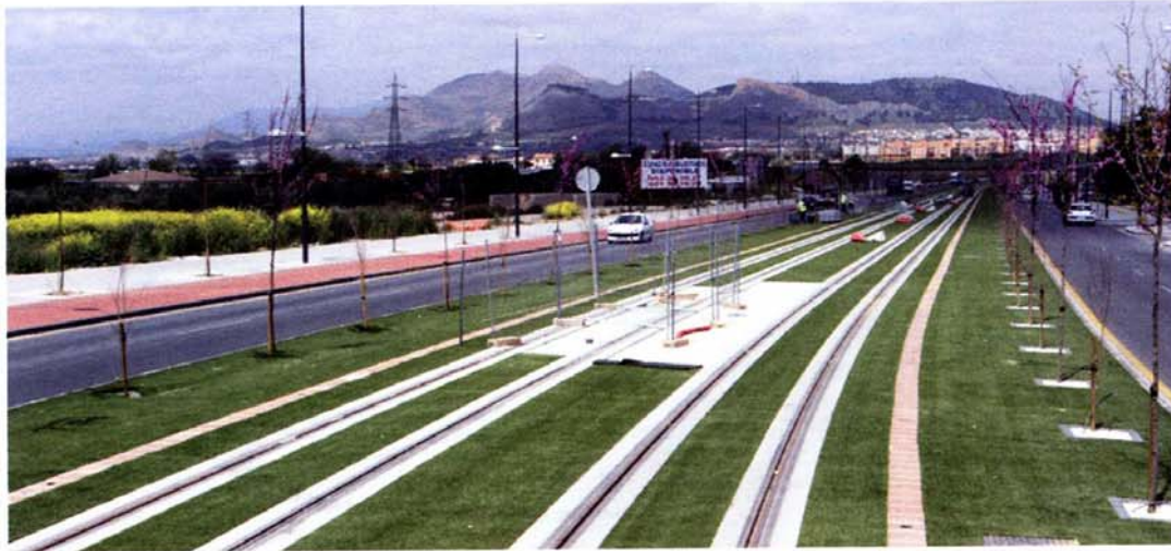
Due for completion in 2012, Granada's 15.9 km north-south line between Albolote and Armilla mainly runs at grade on a reserved alignment.
